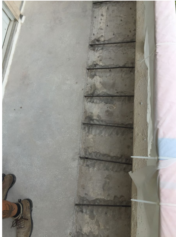
Picture 4: Approved excavation
