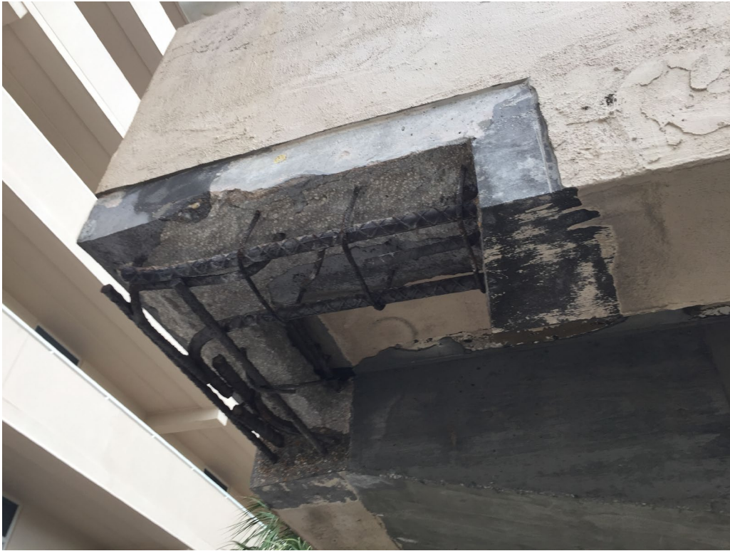
Picture 1: Approved beam excavation
